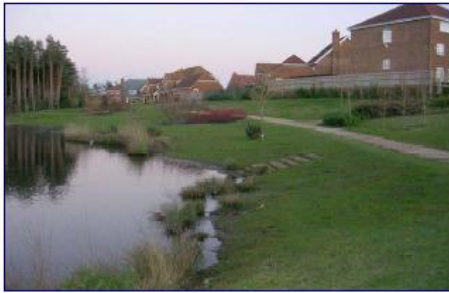
Photo 1. An example of a SUDS pond used to drain a 62ha development at Elvetham Heath
